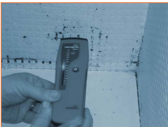
Using a damp meter to assess a damp issue
