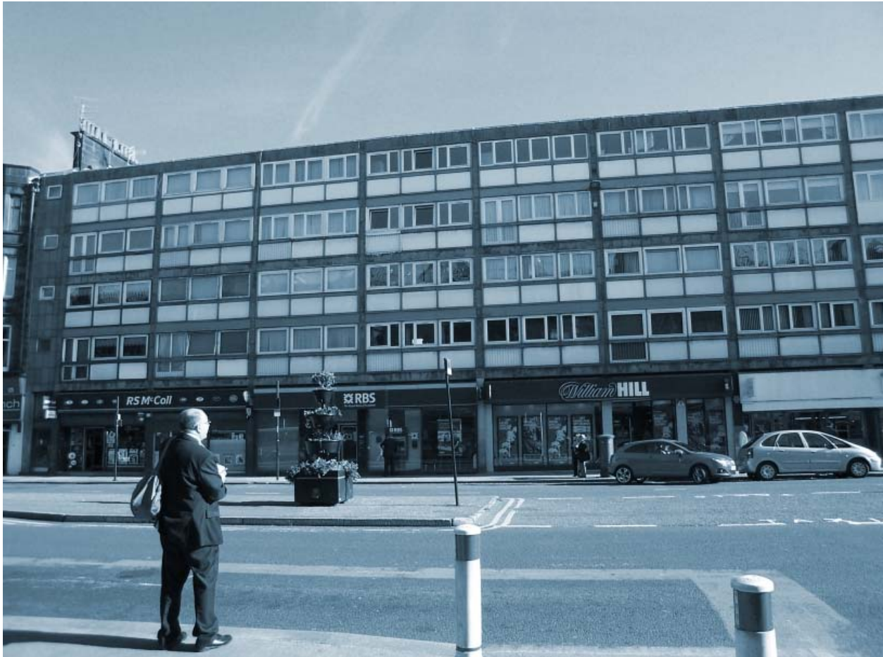
An external inspection of a non-traditional tenement in a rent assessment appeal
